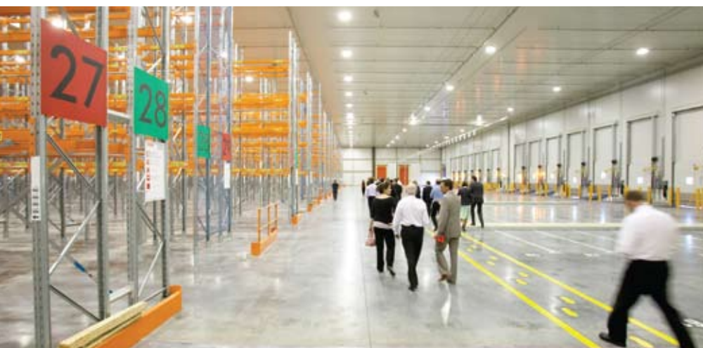
DEXUS Industrial Estate, Boundary Road, Laverton North, VIC
